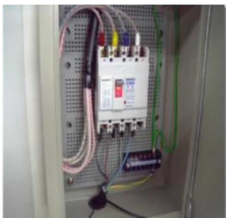
Individual electricity distribution box and a circuit breaker
